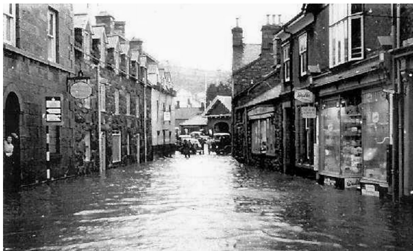
Figure 247: Flooding in Bridge Street, Dolgellau
