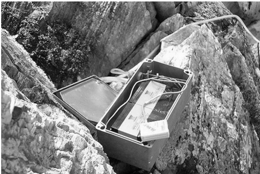
Figure 249: Electronic circuitry, power supply and data logger for the water depth recorder.
